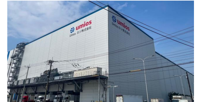
Umios Logistics Corporation, Kawasaki No. 1 Logistics Center
