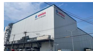
Umios Logistics Corporation, Kawasaki No. 1 Logistics Center
